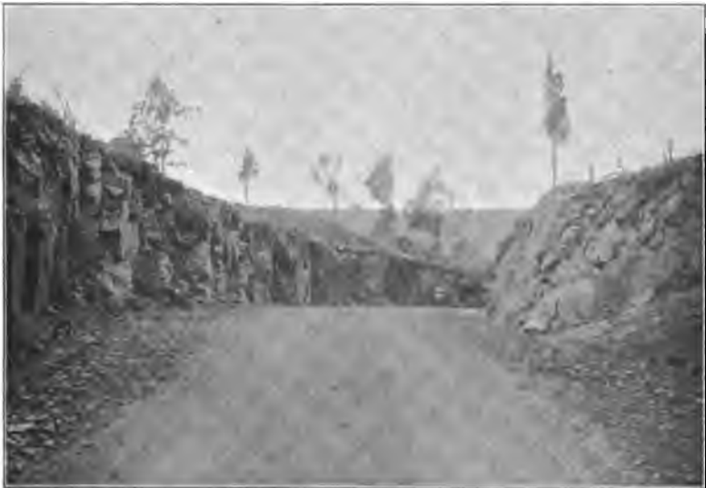
Marshall's Corner and Woodsville road, Mercer Co., showing 15-foot rock cut, after improvement
